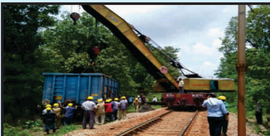
120 T CRANE GROUNDING THE WAGON
