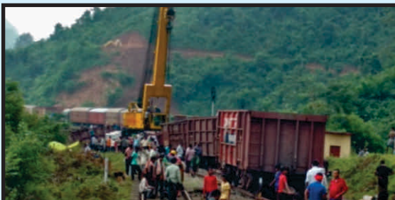
140T BD CRANE IN ACTION AT SKPI
