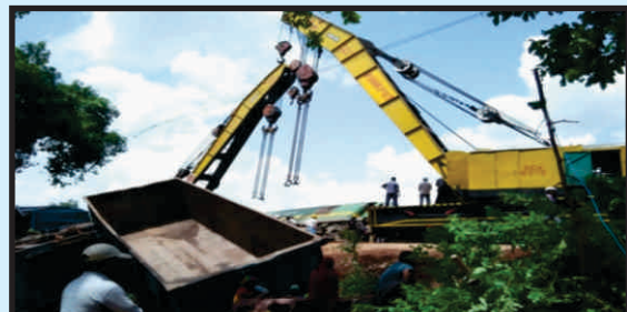
TWO 120T CRANE AT ACCIDENT SITE
